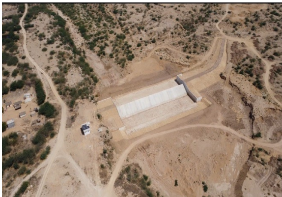
Jharando-1 Dam - Malir
