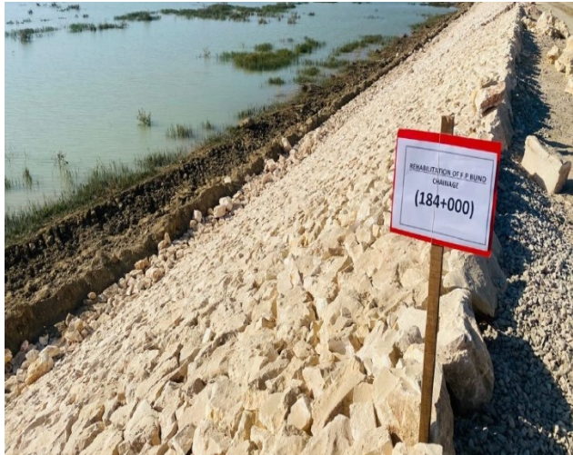
Rehabilitation at F.P Bund
