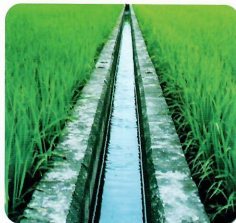
Water Course Improvement
