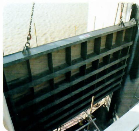
Installation of New Gate Beghari Sindh Feeder Canal
