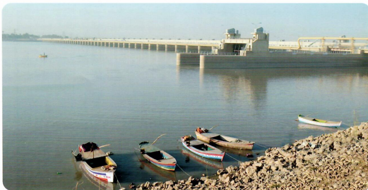
Upstream View of Guddu Barrage
