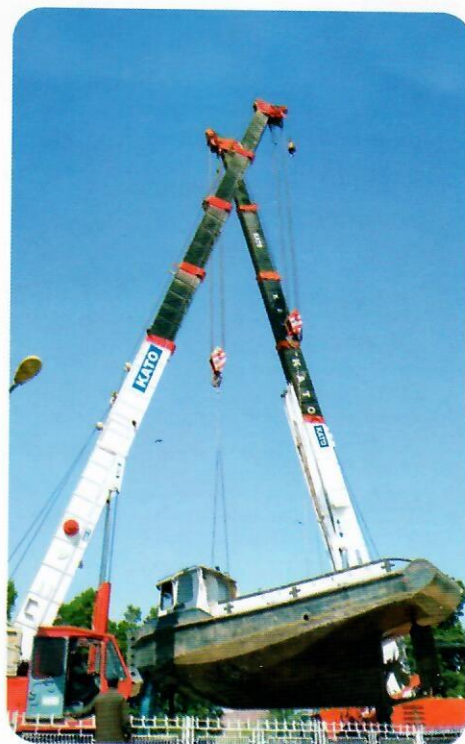
Lifting of Tug for Rehabilitation
